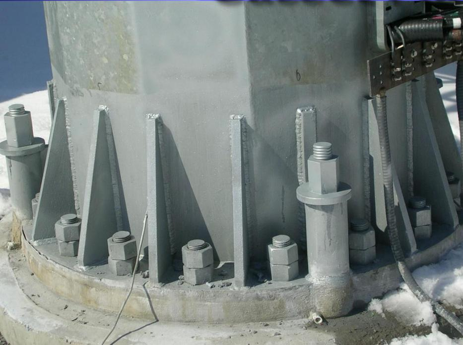
**Base plate reinforcement with 'Tall' gusset plate stiffeners. (Courtesy B. Reese)**
