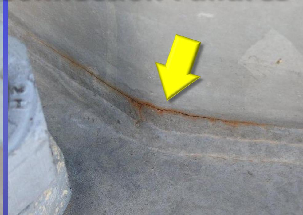
**Toe crack at top of weld at vertex in shaft to base plate connection.**
