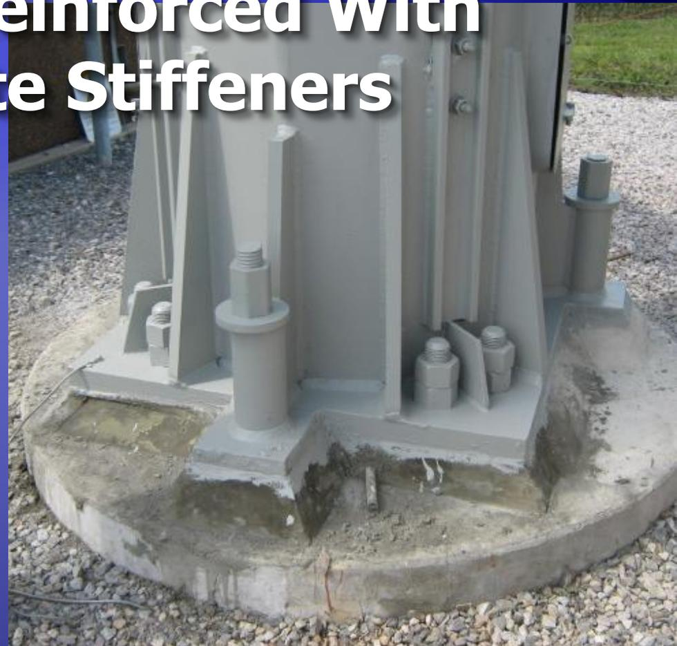
**Base plate reinforcement with 'Tall' gusset plate stiffeners, new anchor rods and brackets. (Courtesy B. Reese)**
